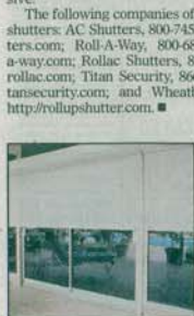
These rolling shutters are partially open over sliding glass doors. Notice the small slotted holes in the flanges between the slats.
